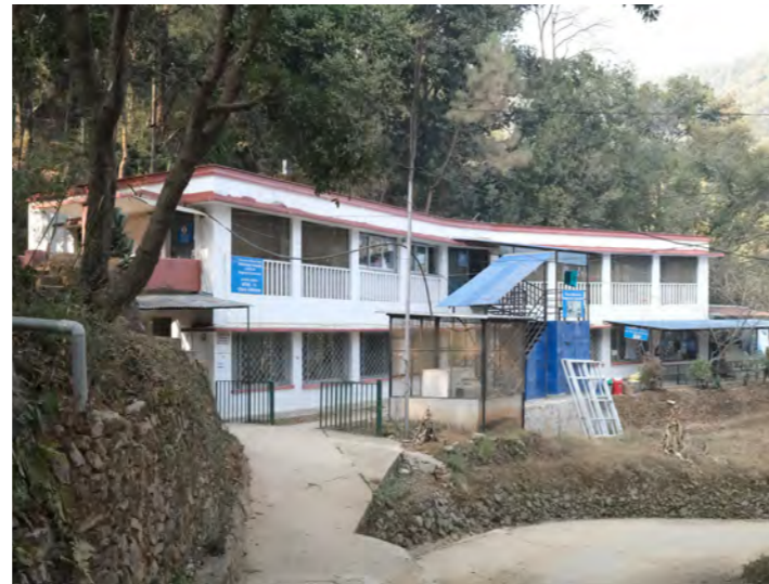
→ The existing laboratory
